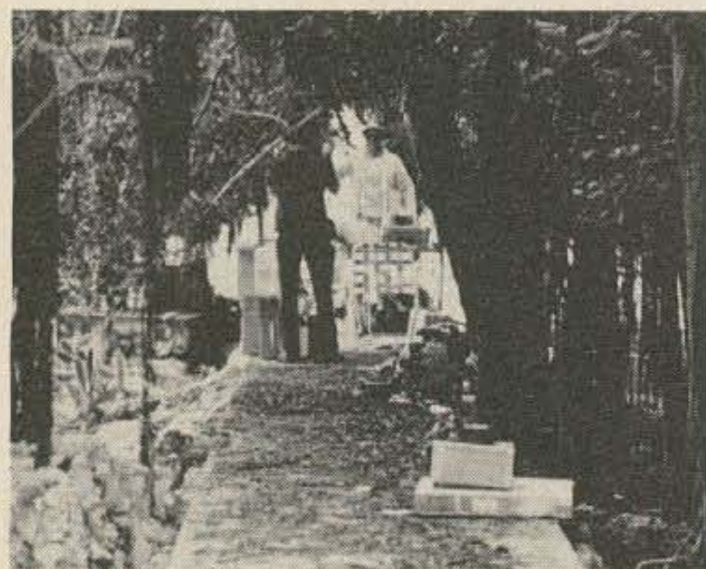
The two generators were set up on a concrete patch that connects the landing area at Lulu Bay and the old Coast Guard acetylene building about 100 yards away. Station number two was set up right near the landing area beyond the generators.
