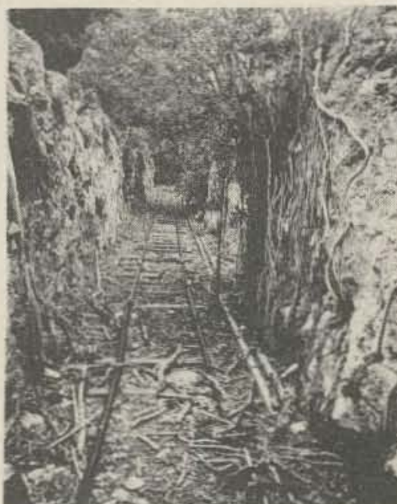
Tracks go along cut about ten feet deep all the way across the top of the island. This facilitated their dumping guano and stuff into the cars from the surface.
