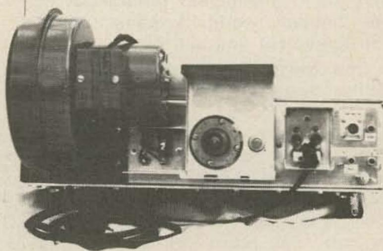
Right to left: Rear view showing ground, alc, H.V. indicator, vox terminals, rf input terminal, ac input showing feed-through capacitor, thyrector and enclosure. Middle enclosure B- and B+ terminals. Left enclosure blower ac supply and fuse. Far left blower.
