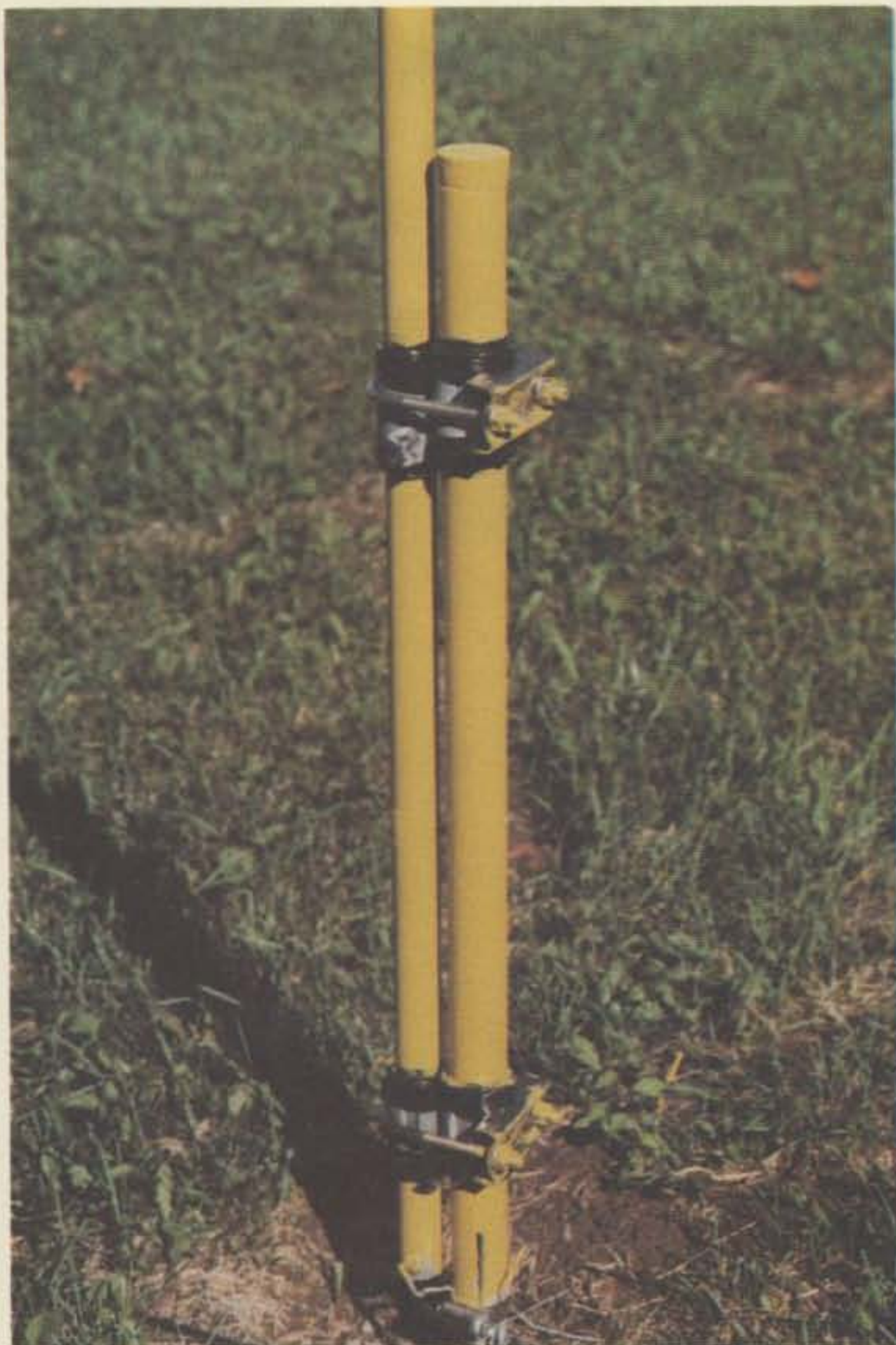
Each of the eight elements is attached to its ground post as shown, using split sections of plastic water pipe for insulators held in place with mylar™ electrical tape and clamped together with TV U-clamps. Refer to Fig. 6.
