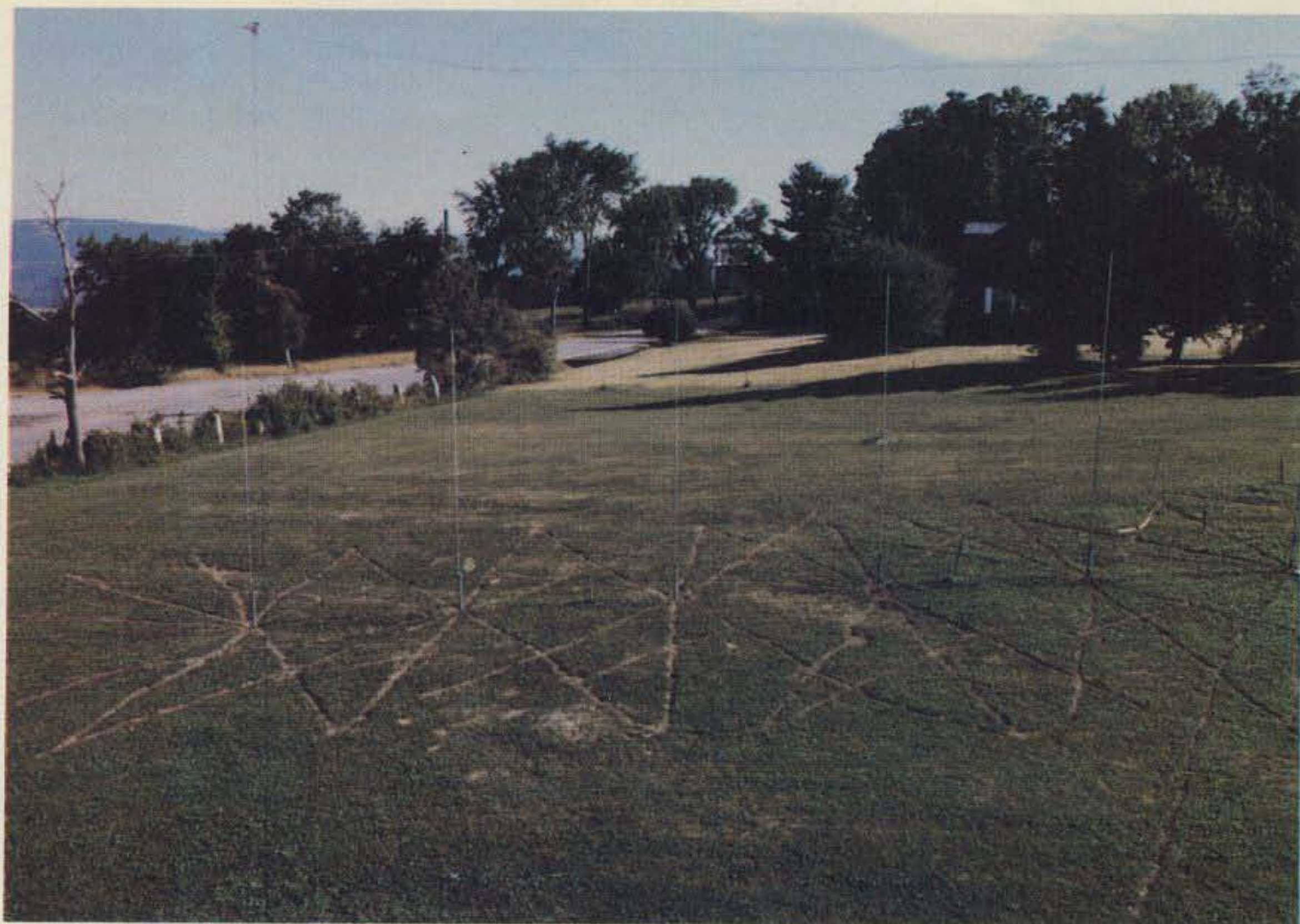
Four more radials were added after this picture was taken, making a total of sixteen; all were from 16 to 20 feet in length. The author employed a trained mole; however, any sharp-pointed garden-weeding or cultivating tool may be used to scratch the shallow trench needed to bury the radial about 1 inch. Refer to Fig. 8.
