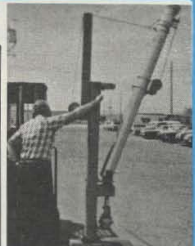
Tilting the tower over is a one-man task with the Wilson bases. (Shown above is the RB-61B. Rotor is not included.)
