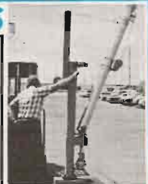
Tilting the tower over is a one-man task with the Wilson bases. (Shown above is the RB-61B. Rotor is not included.)
