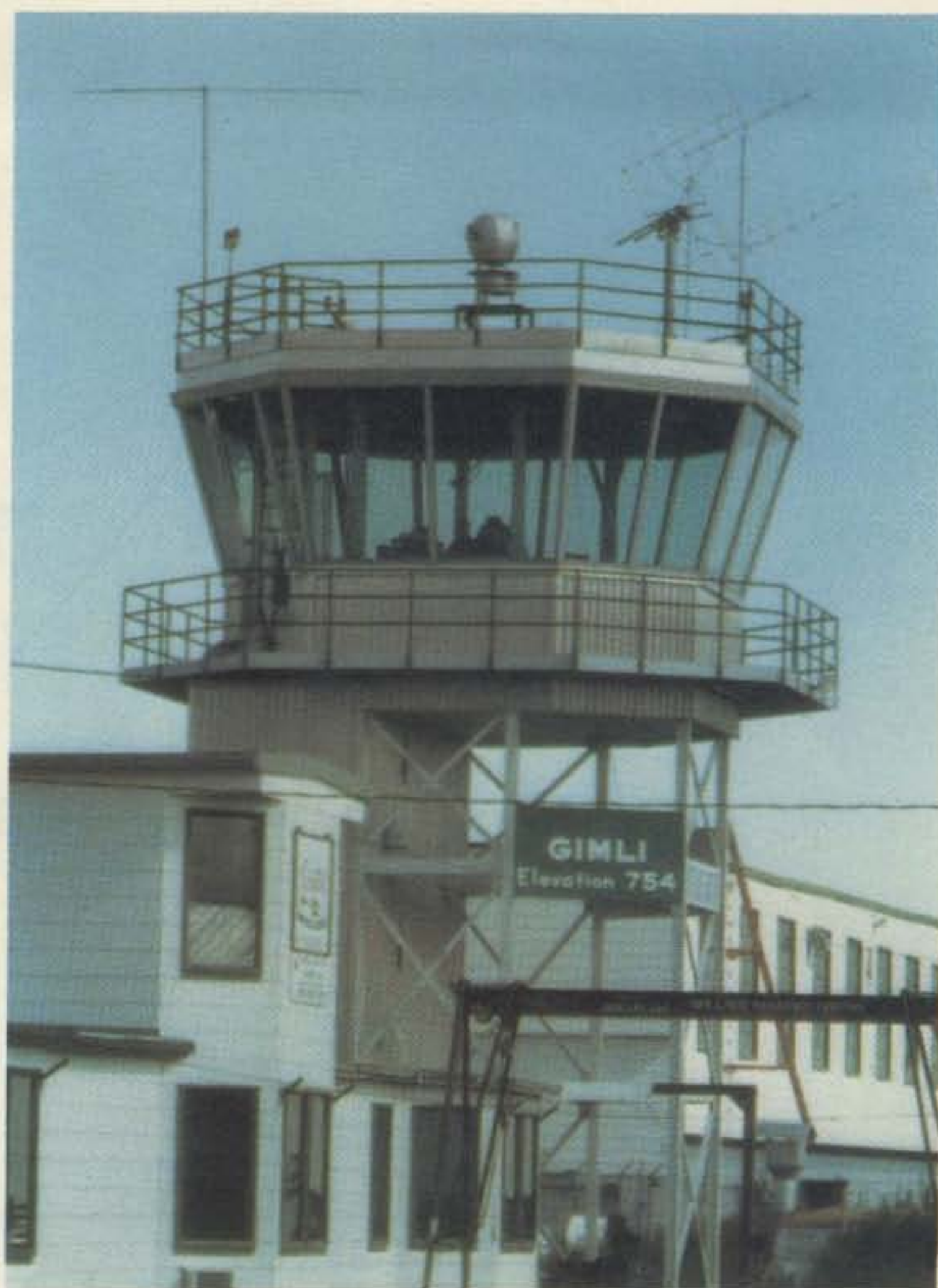
The Gimli control tower. The 4 × 6-element yagi for 2 meters is seen to the right and the 432-MHz beam can be seen to the left.
