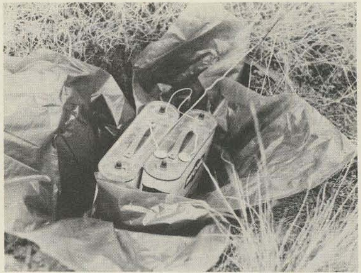
Photo C. The batteries for the transmitter.
