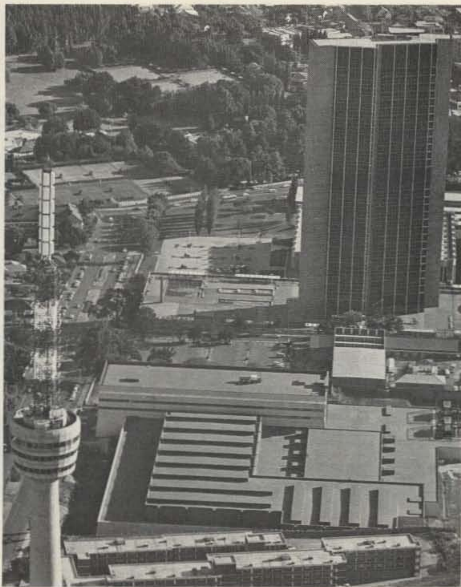
This Johannesburg complex is the home of Radio RSA—the Voice of South Africa. The FM tower is at the left.
