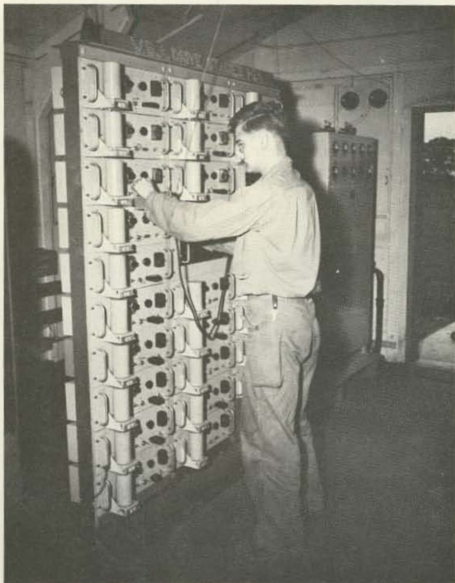
Photo E. The wideband amplifiers were a technical curiosity at Station Charlie, as described in the text.
