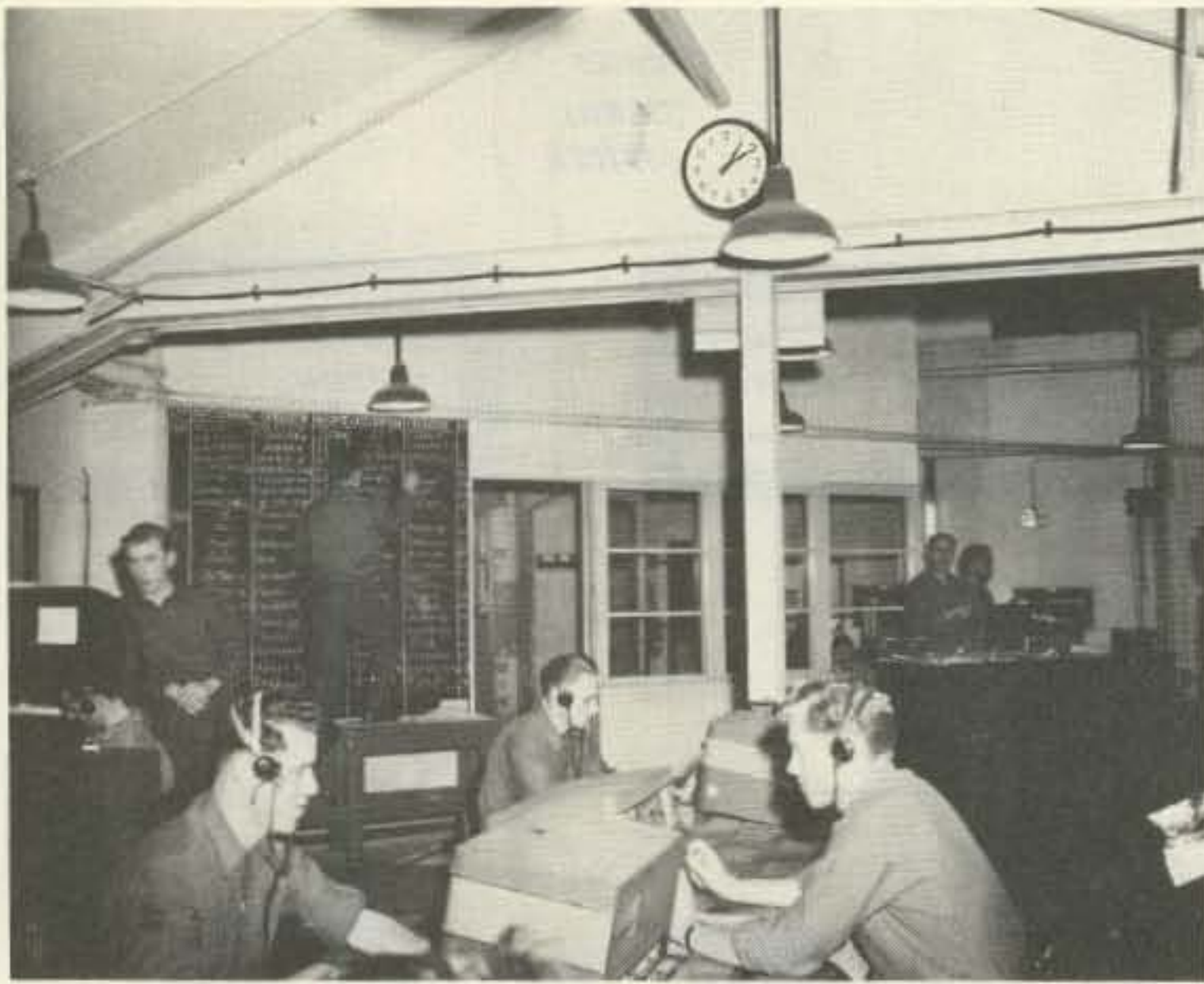
Photo C. A corner of the W/T Room. Agent schedules are posted on the blackboard. The Signalmaster's office behind glass at the rear could monitor any operator position.
