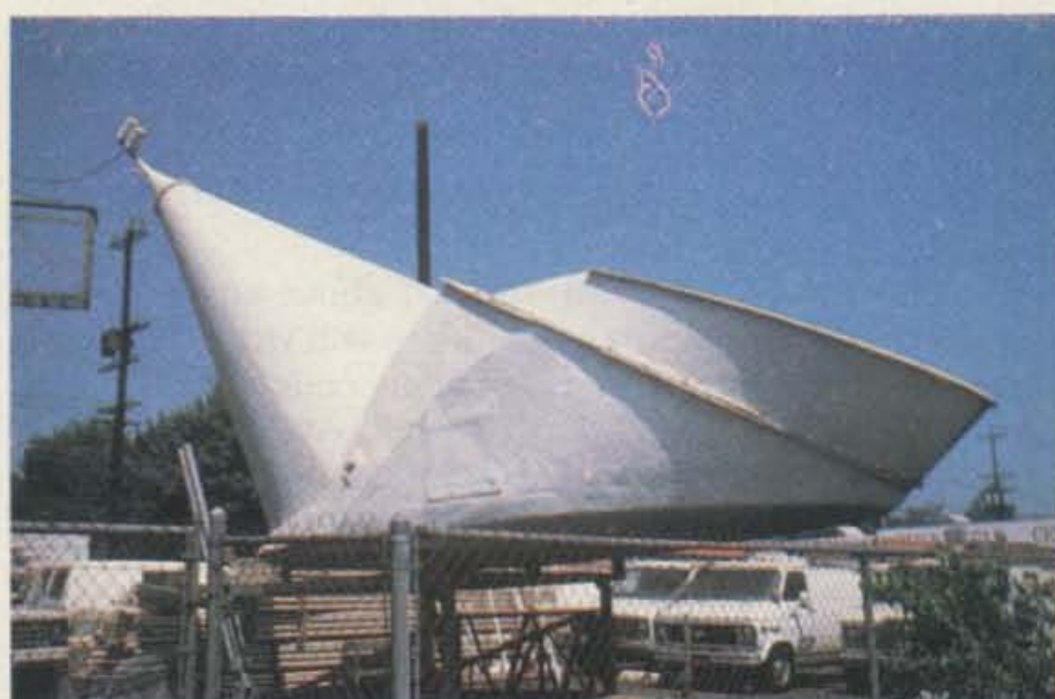
Fig. 4. The horn/reflector antenna is just a segment of a parabola fed by a very long horn. It has been in use for many years by A.T. & T. and other terrestrial microwave users. This design is considered by many as the ideal solution to high gain and low side-lobe response.
