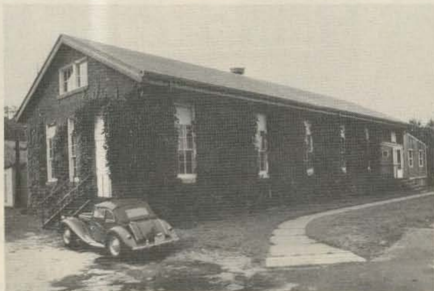
Fig. 2. In this rustic, ivy-covered building with a history as long as radio communication itself, 900 messages a day are handled by 21 professional CW operators, almost half of whom are hams.
