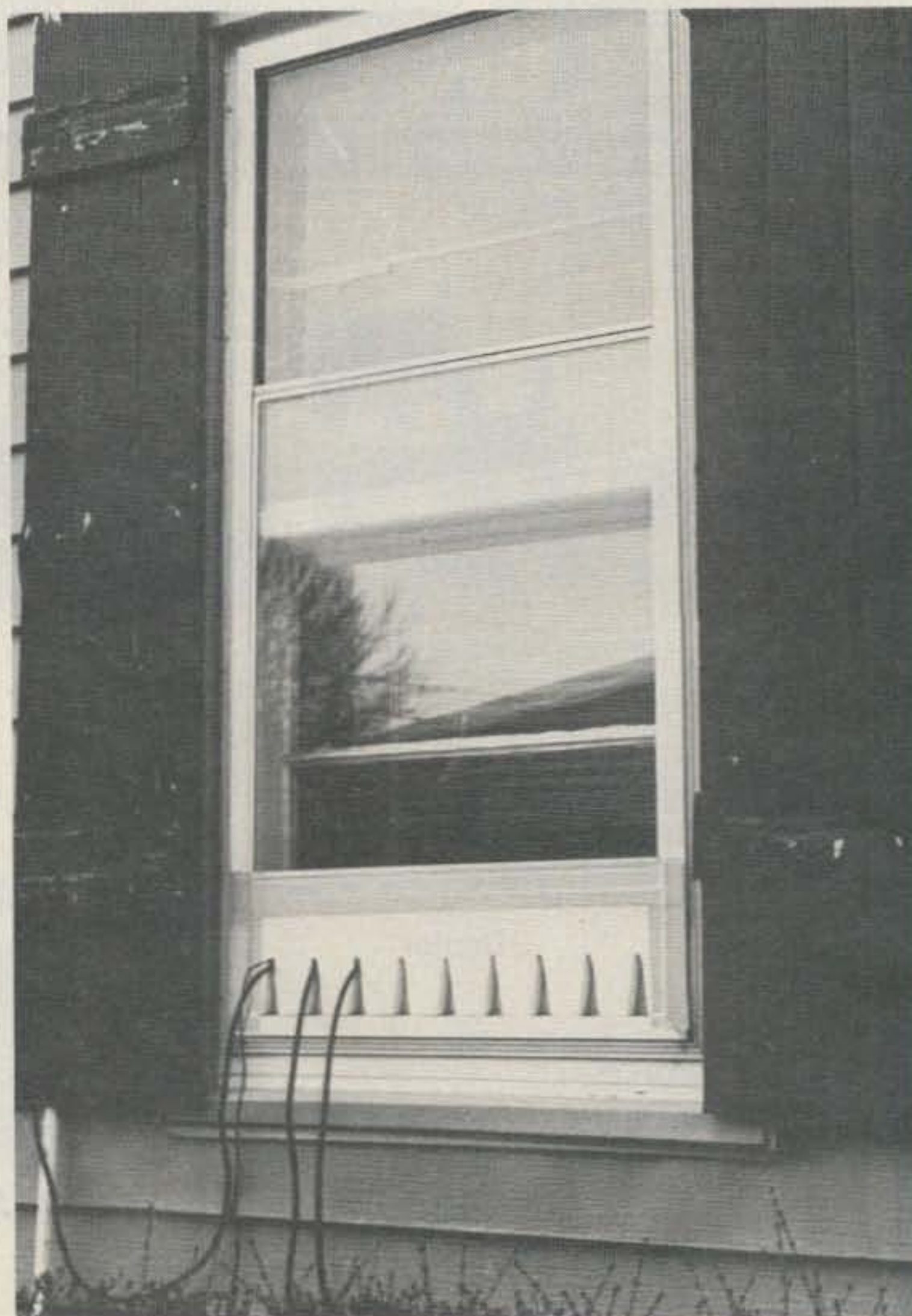
Lines in; window weatherproofed.
