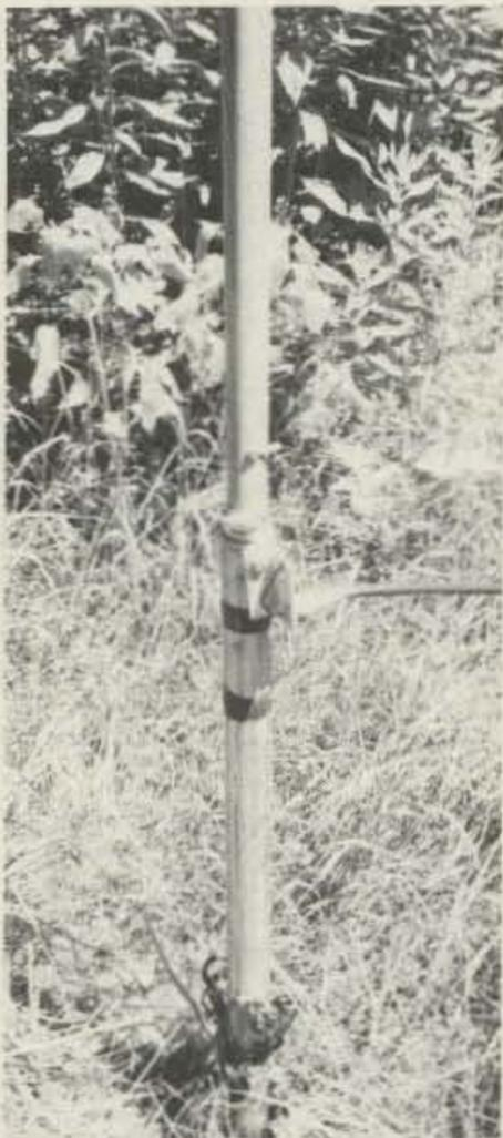
Photo A. The pipe mount is simply sledgehammered into the ground. Note the simple ground system attachment: a long 1/4" #20 bolt with radials soldered into grounding lugs. The two black horizontal stripes are some spare tape left on the pipe.
