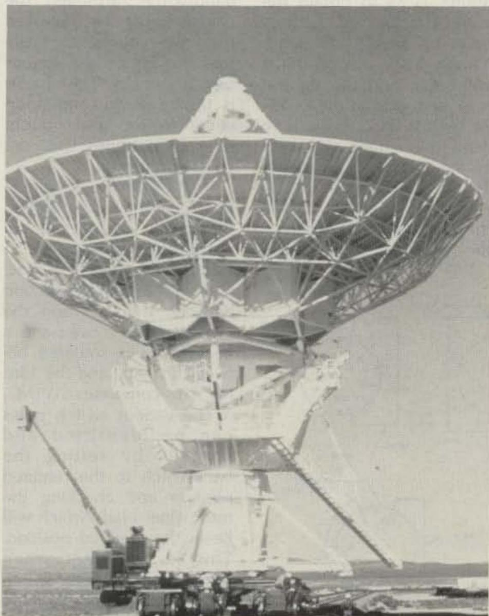
*VLA antenna on the rail transporter which is used to move the antennas from one site to another.*
