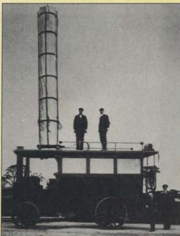
The smokestack-shaped structure on the car roof is the first mobile antenna, invented by Guglielmo Marconi in 1897. It was soon replaced by the more modern "clothesline" antenna (so named because it looked like six lengths of clothesline strung between poles at the front and back of the car). The familiar whip antenna came on the scene only in 1937.
