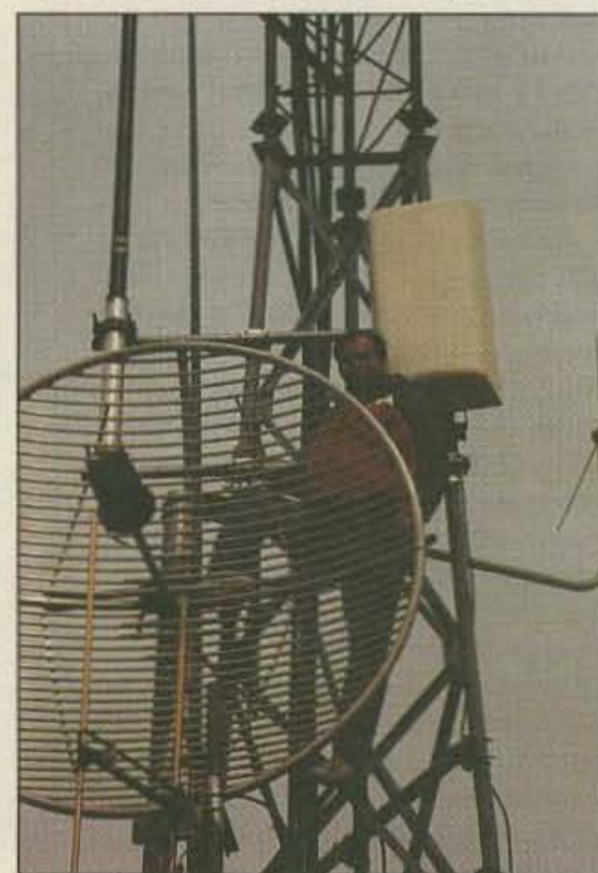
Photo C. Geoff KB7BY adjusts the 23cm antenna which helps link the Mt. Potosi, Nevada ATV repeater into Los Angeles.
