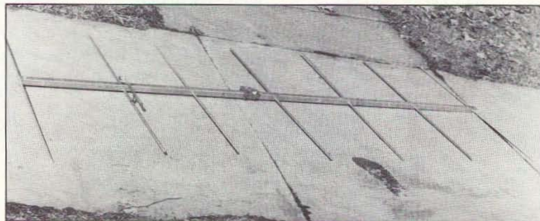
Photo E. The completed beam.
