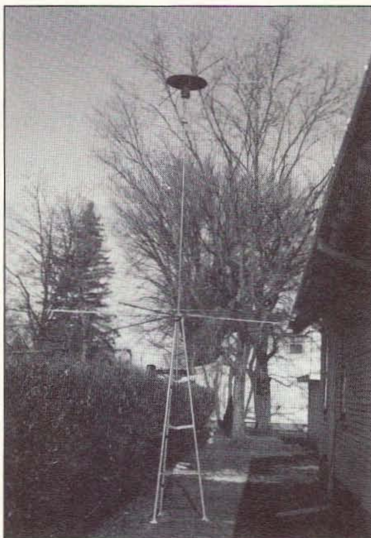
Photo A. The discone.
