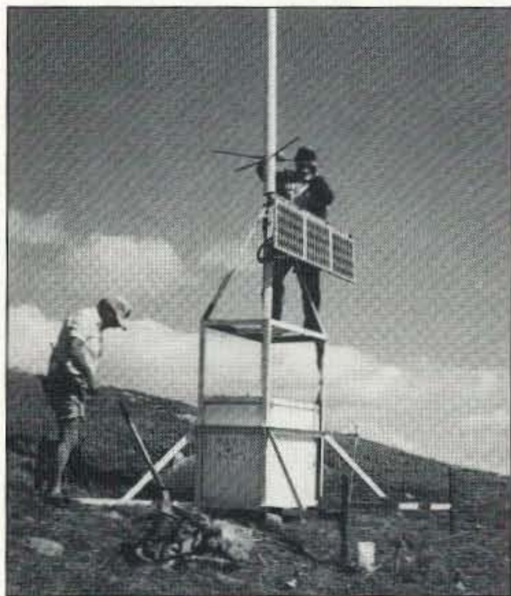
Photo E. VE7HRC (on ground) and VE7EMS (atop the unit) work on the "solar lander module."
