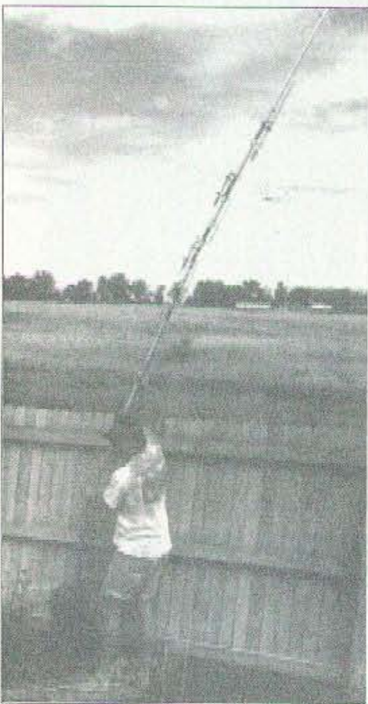
Photo B. KBØSJX positioning his antenna so that it may be dropped over a pipe driven into the ground at the rear of his fenced-in property. The coaxial cable from his shack meets up with the antenna and the "instant antenna-raising ceremony" is complete.
