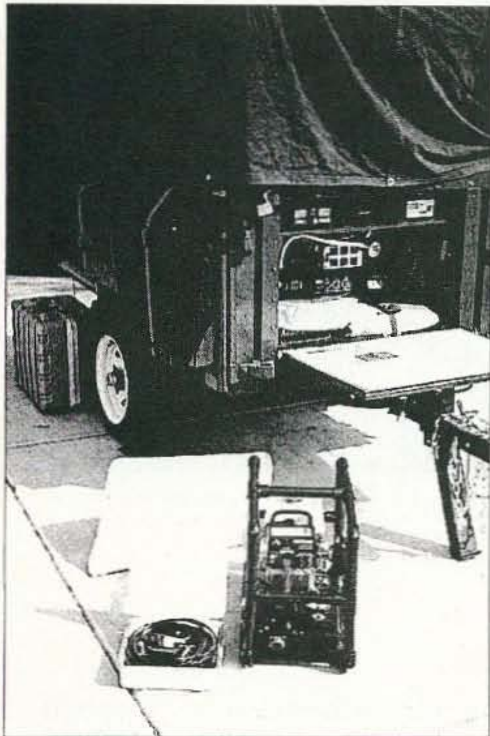
Photo E. Genset and DC cable set for battery recharge.
