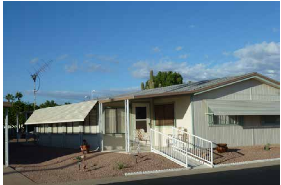
Figure 1: Showing the antenna system relative to the home. The idea was to make this blend in with other TV antennas. Antennas are 15' above the ground and about 3' above the roofs.
