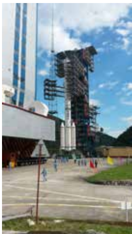
Figure 9: Removal of the launch tower.
