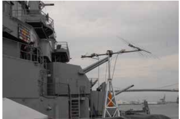
Photo 7: NI6BB satellite antennas installed aboard the Battleship Iowa
