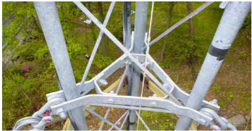
Figure 4 — Guy bracket [Courtesy www.w3yy.com/Phillystran.htm .]
