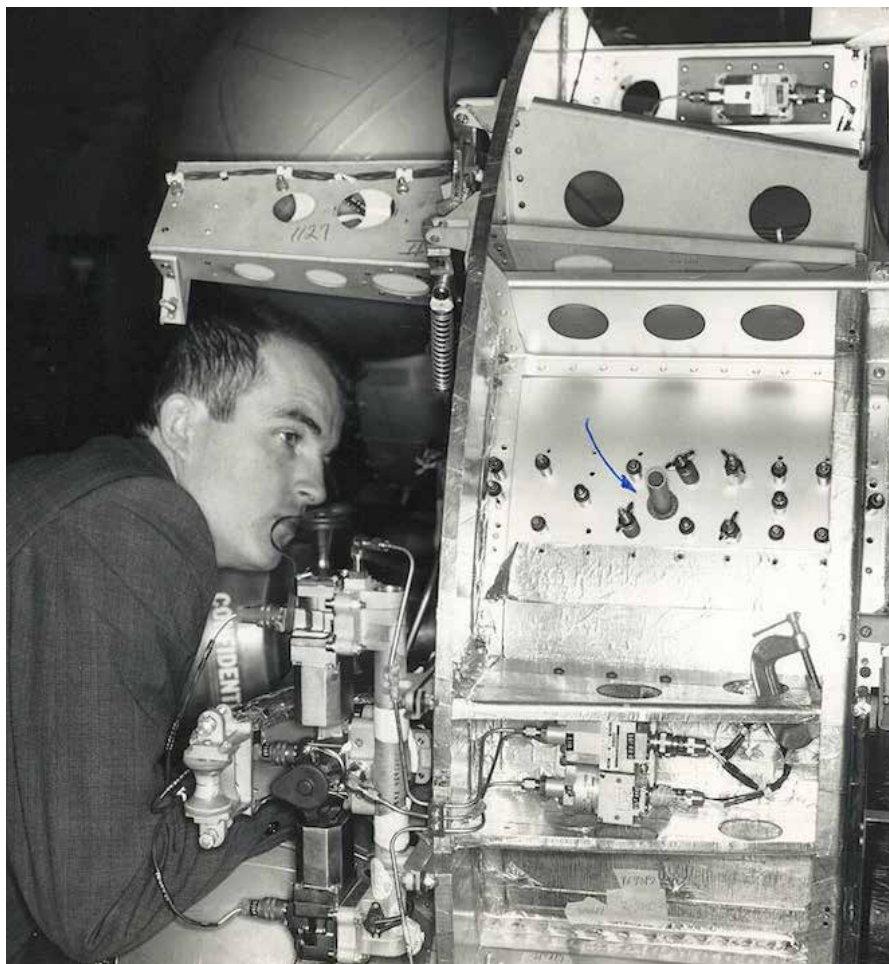
Lance Ginner inspecting OSCAR 2 ejection mechanism (Courtesy: AMSAT).
