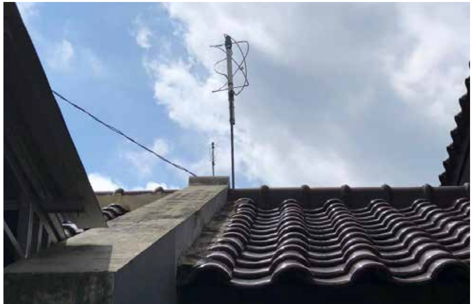
Figure 9 — QFH antenna used by YD2UUY.
