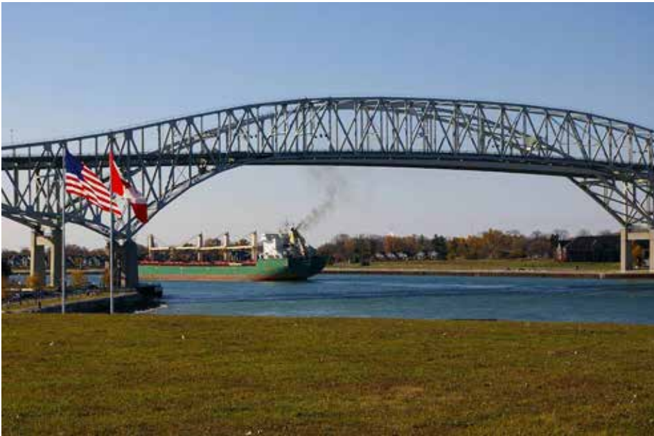
The international Bluewater Bridge between Port Huron, Michigan and Point Edward, Ontario (near your author's home) forms the second busiest land border crossing between Canada and the United States. (KB1SF, photo.)
