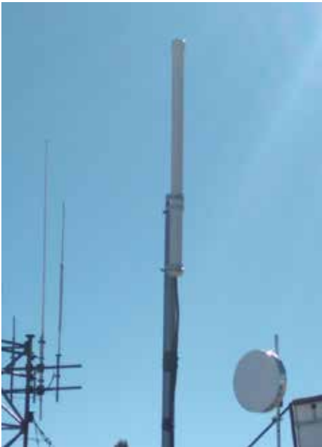
Figure 16 — A 400-435 MHz sleeve dipole at the Toro Peak repeater site in southern California, elevation 8717' (2657 m).
