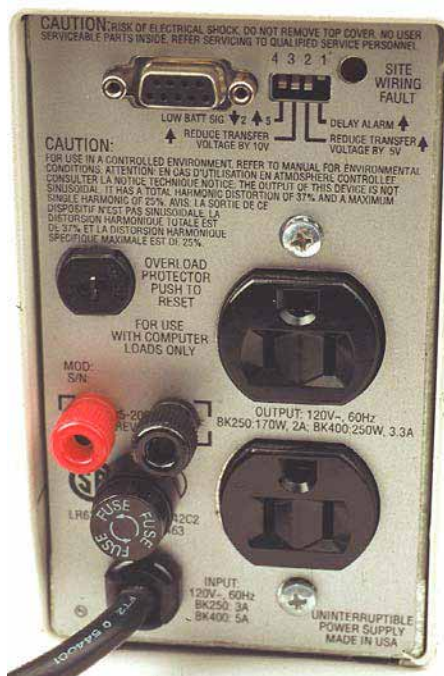
Fig 17.53 — This rear-panel view of a converted UPS shows a pair of binding posts for the 12 V dc connections and a fuse holder for the 12 V output. Carefully position and drill the mounting holes for the binding posts and fuse holder, so that you don't damage existing parts. Ensure that the placement of these parts will not interfere with any existing components. A Unibit or KWIK STEPPER is ideal for cutting through the 1/8-inch thick steel rear panel. (See "Tool Tips," Technical Correspondence, QST, Dec 1998, p 63.)
