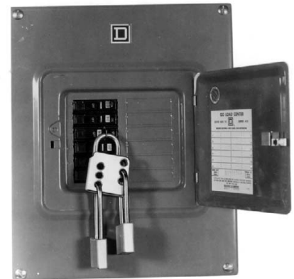
Fig 3.2 — If the switch box feeding power to your shack is equipped with a lock-out hole, use it. With a lock through the hole on the box, the power cannot be accidentally turned back on. (Photo courtesy of American ED-CO)
