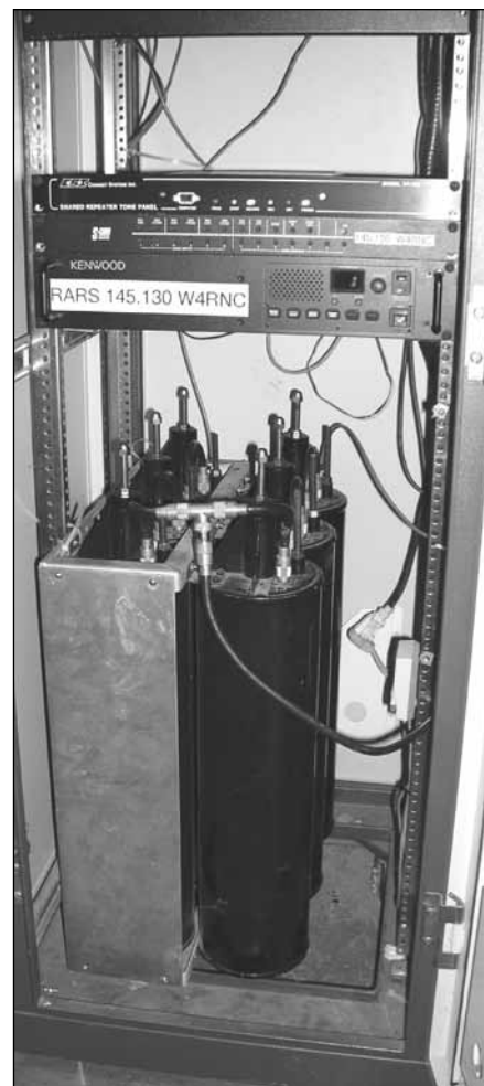
Fig 18.6 — The W4RNC 2-meter repeater includes the repeater receiver, transmitter and controller in the rack. The large object underneath is the duplexer. (photo courtesy KN4AQ)
