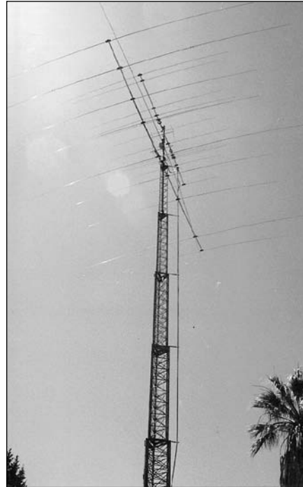
Fig 28.11 — The bottom of N6TV’s crank-up tower is shown at left. The motor drive mechanism is on the left and a fishing net on the right catches and coils the feed lines and control cables as the tower is lowered. On the right, K6KR’s fully loaded crank-up extended to its maximum height of 90 feet. (K7LXC photos)
