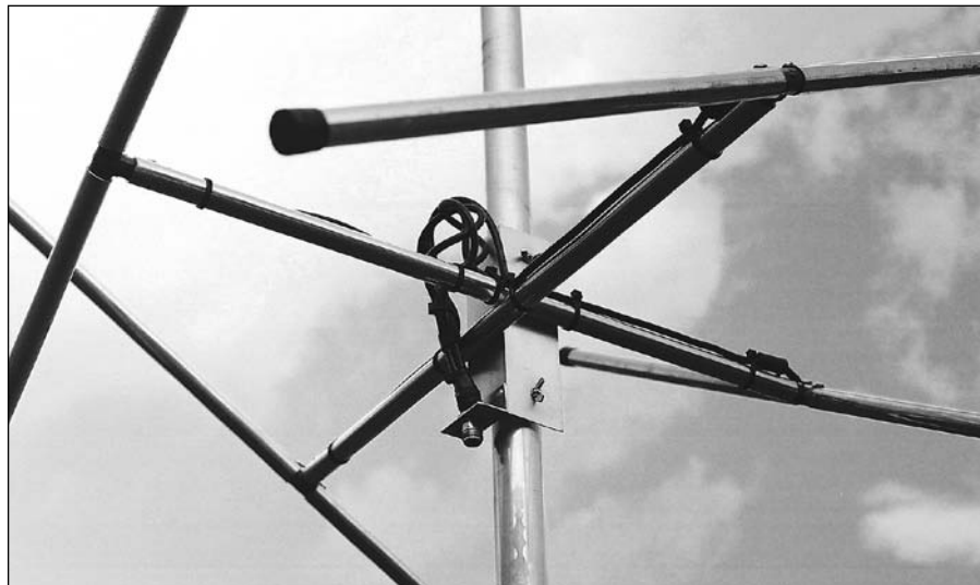
Fig 47 — View of cross booms mounted to mast.
