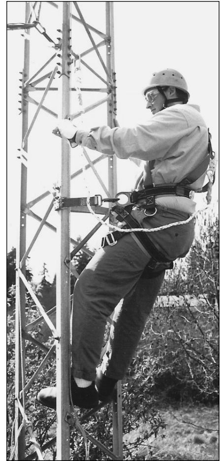
Fig 28.21 — The fall-arrest lanyard is above the climber so that the climber can climb up to it. The fall-arrest and positioning lanyards are then "leapfrogged" so that the climber remains attached to the tower 100 percent of the time. (K7LXC photos)
