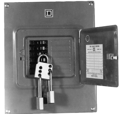
Fig 28.2 — If the switch box feeding power to your shack is equipped with a lock-out hole, use it. With a lock through the hole on the box, the power cannot be accidentally turned back on. (Photo courtesy of American ED-CO)
