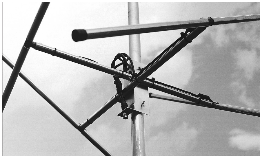
Fig 47 — View of cross booms mounted to mast.
