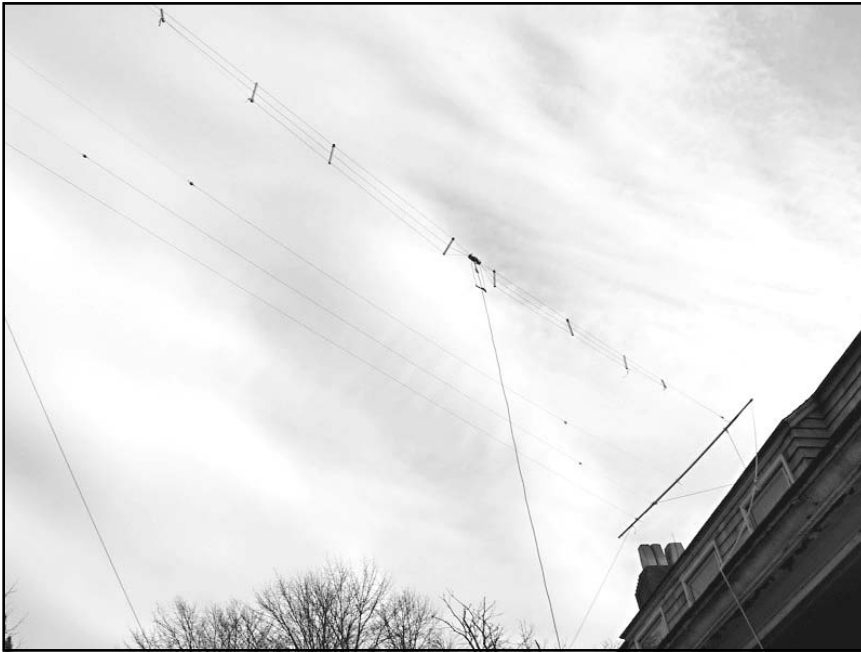
Fig 33 — VE7CA portable 2-element 20/15/10-meter wire Yagi installed at Plimoth Plantation in Plymouth, Massachusetts. (Photo courtesy K1HTN).
