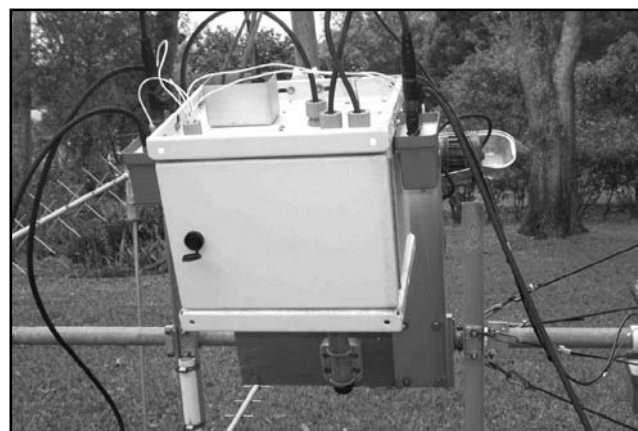
Fig 61—A NEMA4 box is used to shelter the L-band electronics and power supply. The box flanges are convenient for mounting preamplifiers. The box is shown inverted since it is on a tilt-over tower. (WD4FAB photo.)
