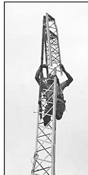
**Fig 22—Climber is guiding the new section onto the top of the existing one. The gin pole attached to the left leg is bearing the weight, as the climber gives verbal instructions to the ground crew pulling on the gin-pole rope. (Photo courtesy Mike Hammer, N2VR.)**
