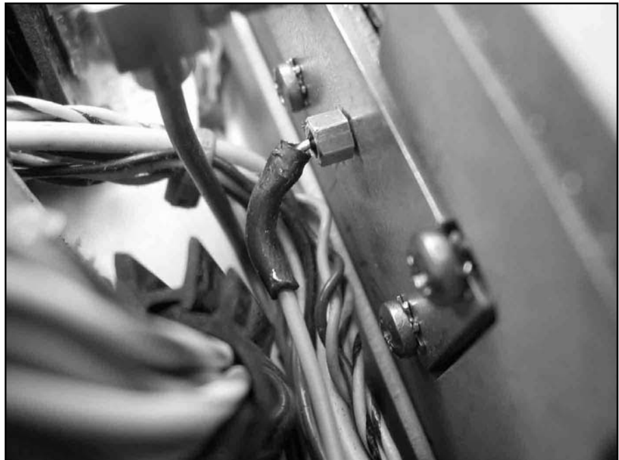
Fig 2—Detail of added feedthrough insulator.
