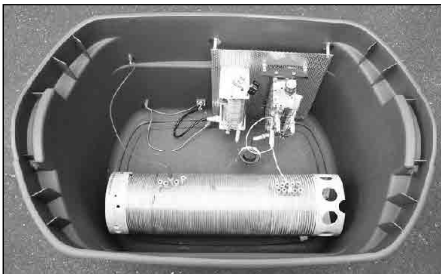
Photo B — This is the 500-kHz antenna tuner used at the author's station, WD2XSH/14.
