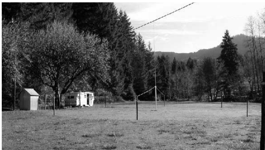
Figure 3— A view of the test antenna area and test equipment shelter. The receiving antenna is at the far end of the pasture.
