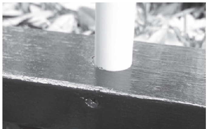
Figure 11 — PVC pipe secured to the TASH antenna base by a wood screw.
