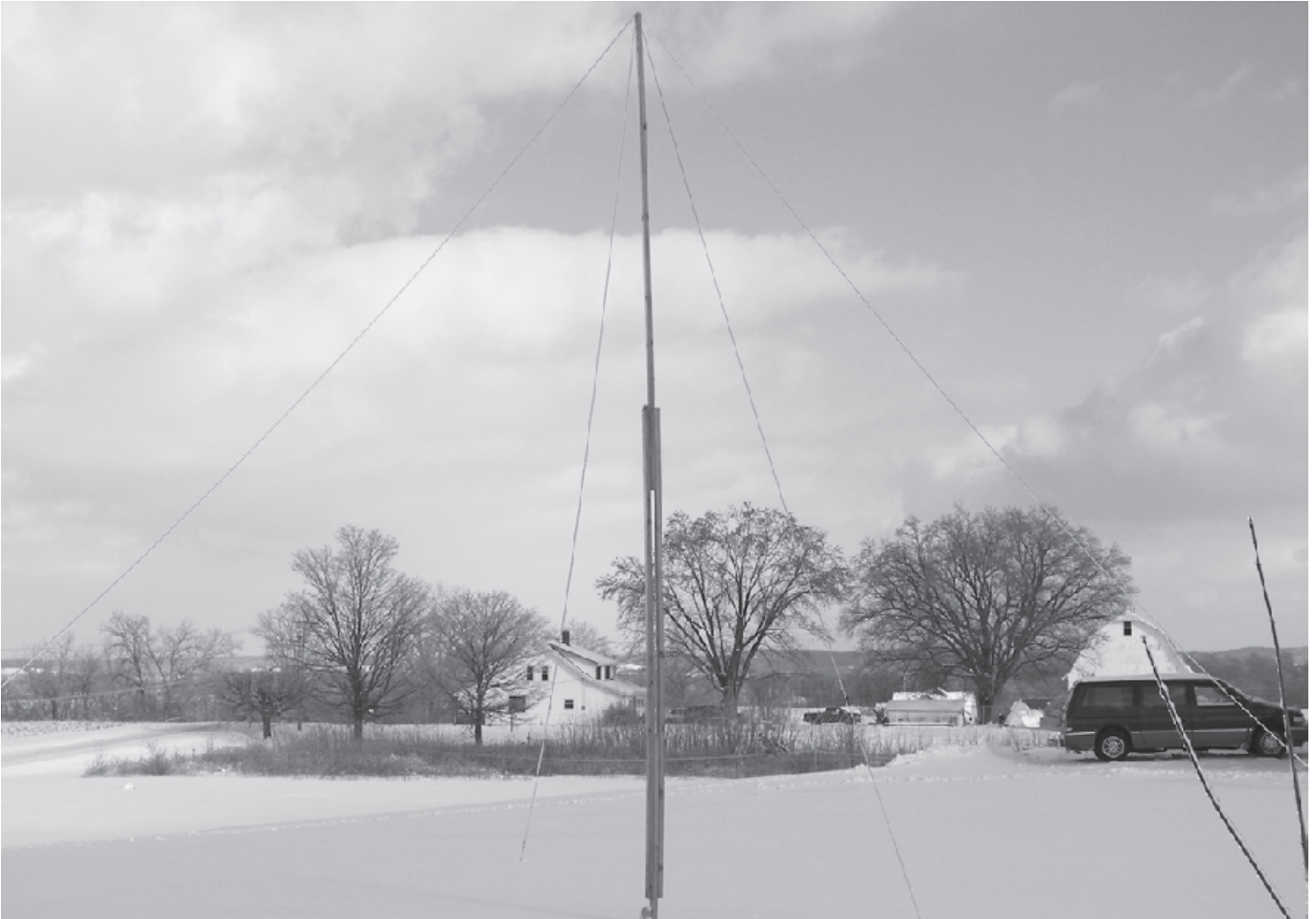
Figure 10 — One way to build a short vertical. This antenna consists of three 12 foot 2x4s screwed together with deck screws so that the bottom two 2x4s overlap the top 2x4 by 2 feet. The bottom 2x4s are mounted 1 foot high on a bolt through an 8 foot 2x4 buried in the ground so that the overall height is 23 feet. An AWG no. 10 copper wire runs the length of the 2x4s and joins four 23 foot top hat wires that also guy the structure. The 2x4 buried in the ground provides extra rigidity so that the vertical is less likely to break in the middle, as the first several did. Ice on the top-hat wires enhances visibility.
