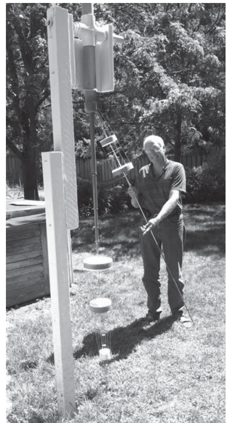
Photo 1 — N6GN holding a bottom launcher and pointing toward a second launcher installed at the base of the All-Band HF /VHF/ UHF antenna. The PVC tilter can be seen in this Photo. Styrofoam doughnuts have been added to keep the center conductor concentric with the outer cone.
