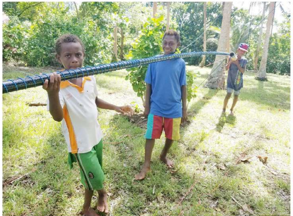
Figure 1 — The vertical radiator spiral-wound inductor windings are spaced 1.4 inches. We got local help to construct and erect the antenna.
