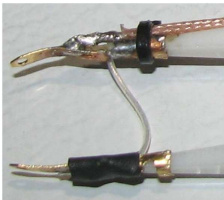
Figure 6 — Cable connections to spade lugs with strain relief.
