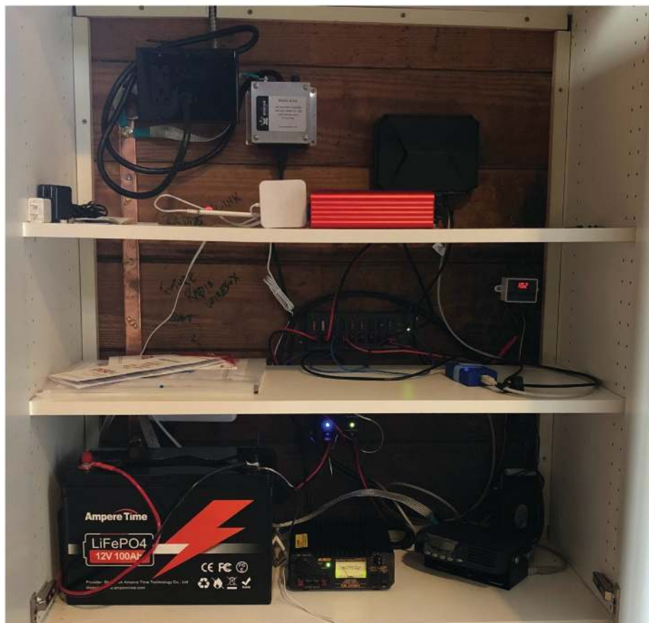
Photo 13 — The completed station with room for storage and expansion.
