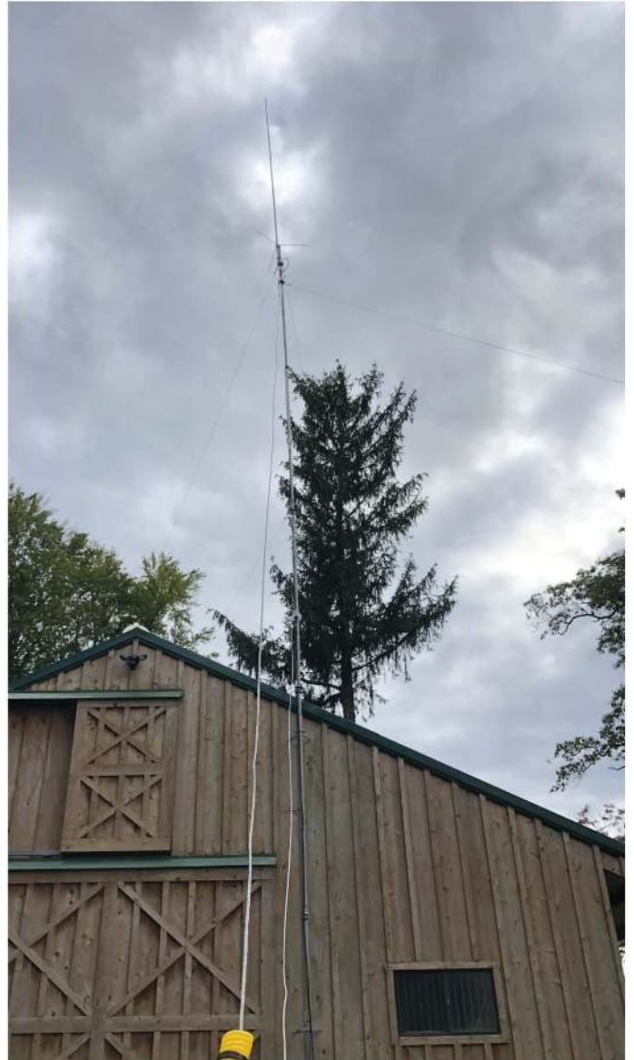
Photo 9 — “Antenna back up” two hours later. The narrow barn hadn't allowed for enough spread for three point guys, so a fourth point at an approximately right angle to the barn peak trued up the mast.
