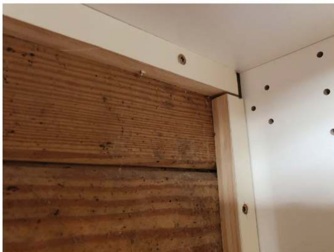
Photo 2 — Detail of cabinet attachment to barn wall.
