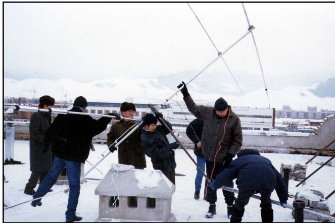
Fighting -35° temperatures, the iron men made it but their coax did not. The plastic insulation of RG8X broke into pieces. We were way out of temperature specs for this cable.
