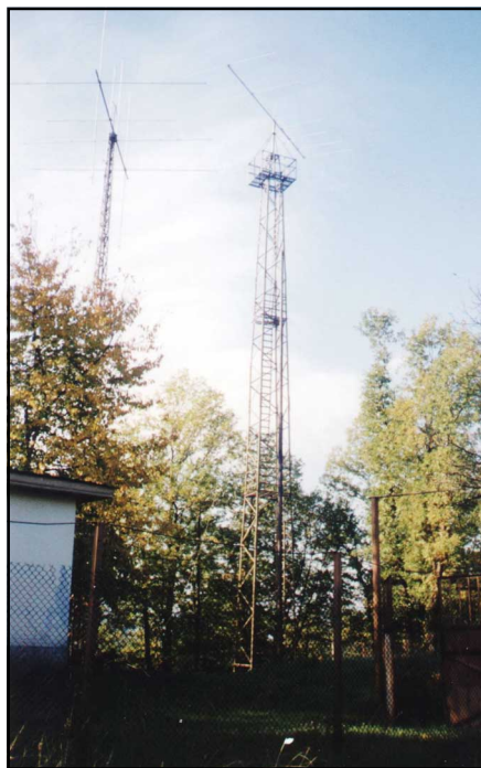
The quad at LZ9A is 3 elements on 20 meters and 4 elements on 15 and 10 meters. The second tower supports a 6-element 10 meter Yagi.
