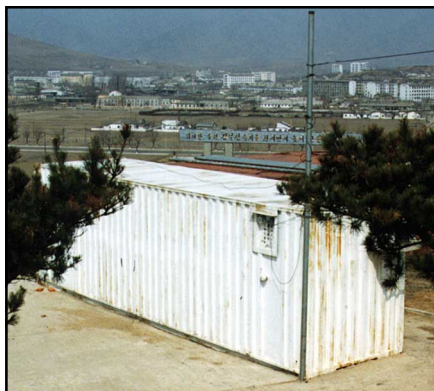
P51BH signals emanated from this structure overlooking the city of Rajin. It housed a telecom cellular base station soon to serve the city below. Cables were run up a 120-foot tower.
